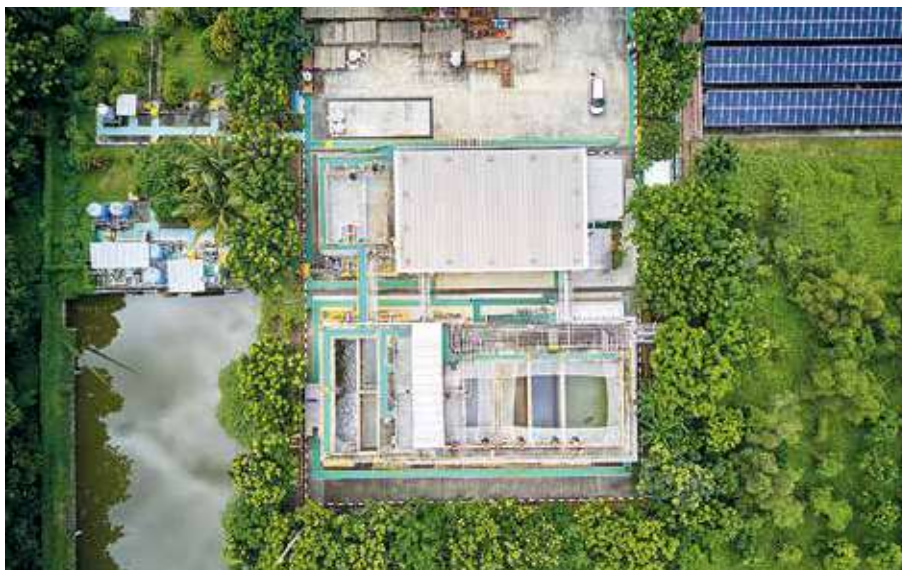
Instalasi pengolahan air dan solar panel di pabrik Karawang 3. Water treatment plants and solar panel at Karawang 3 factory.
